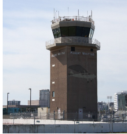
Airport Traffic Control Tower
