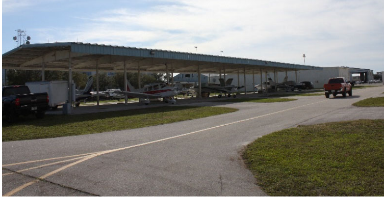
SPG Shade Hangars
