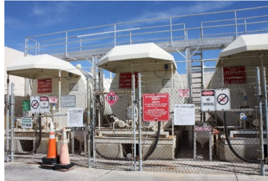
Airport Fuel Farm
